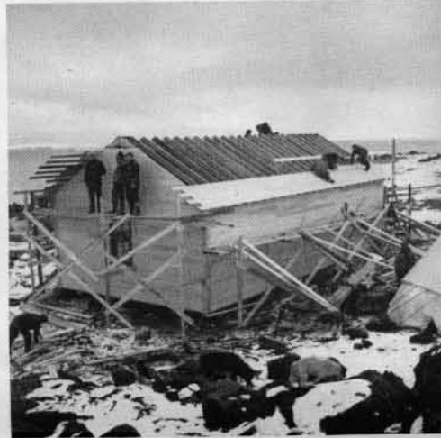
Construction of Fort Ross; the warehouse. Every-body digs in.
