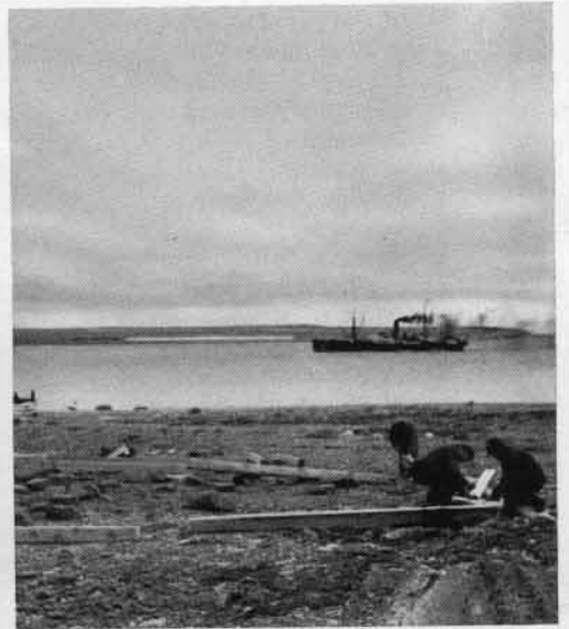
Laying the foundation for Fort Ross.
